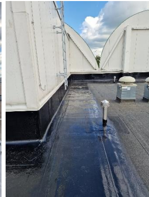
polyurea on bitumen
