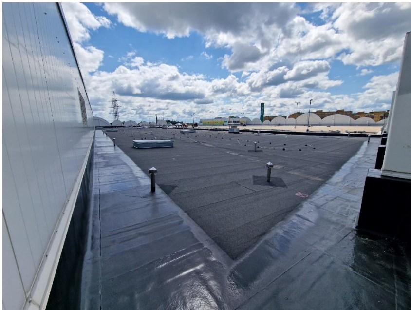
Teknos Teknopur polyurea system for the concrete slab and bitumen membrane (flat roof).
